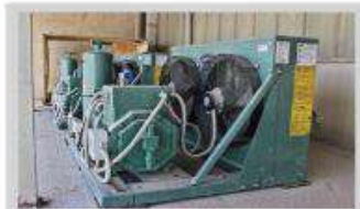
Individual condensing unit (semi-hermetic & hermetic)
